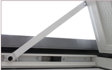
Door closure with integrated locking system
