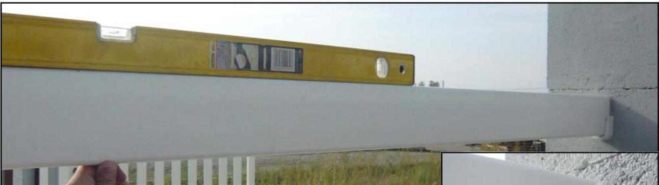
Using the Rail, position the support of the opposite bottom part so that it is level with the other support. Draw a marker.
