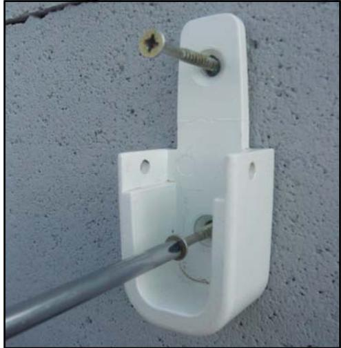
Position one of the supports of the bottom part on the post. Mark the drill holes. Drill, then secure with pins (not provided). Attach the support of the bottom part to the post (screws not provided).
