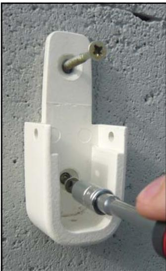
Mark the drill holes. Drill, then secure with pins (not provided). Attach the 2nd support of the bottom part to the post (screws not provided).
