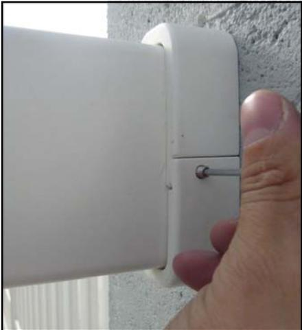
Attach the Rail using the hollow hex screws M5x8, until pressurized. These screws enable the support to be locked in place.
