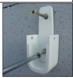
Position one of the supports of the bottom part on the post. Mark the drill holes. Drill, then secure with pins (not provided).
